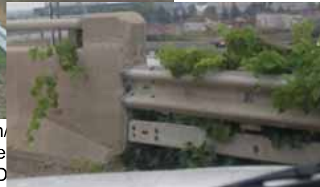
Approach/Leaving End Treatments: Bridge
